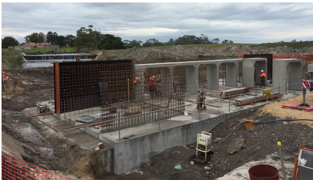
Figure 3. The new Blackford Drain regulator under-construction
