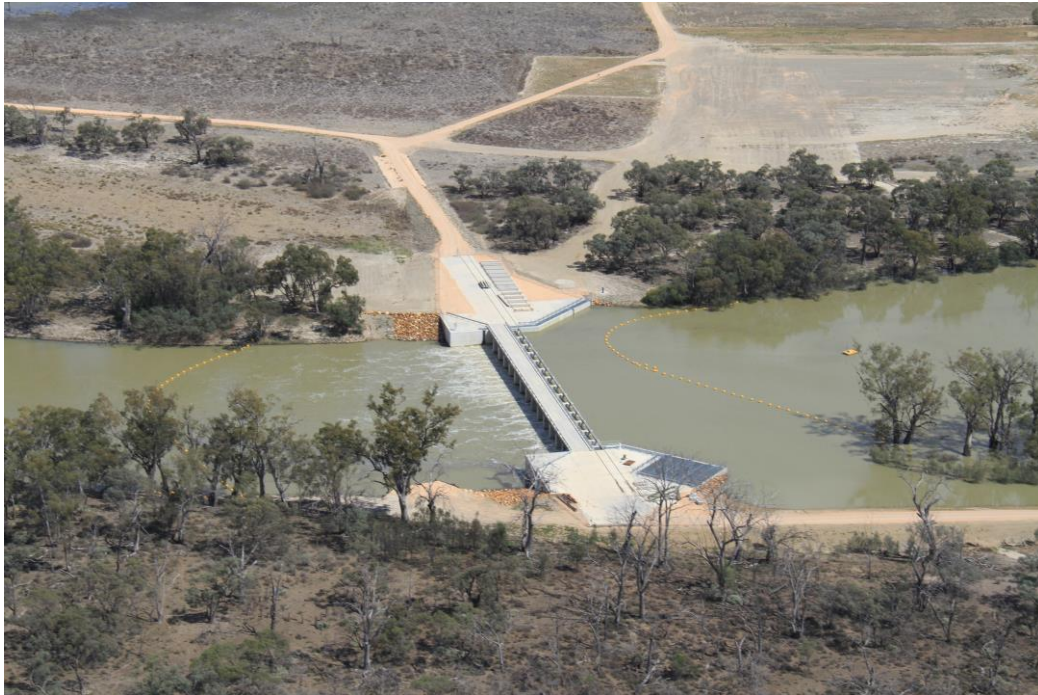
Photo: Chowilla Creek environmental regulator in operation
