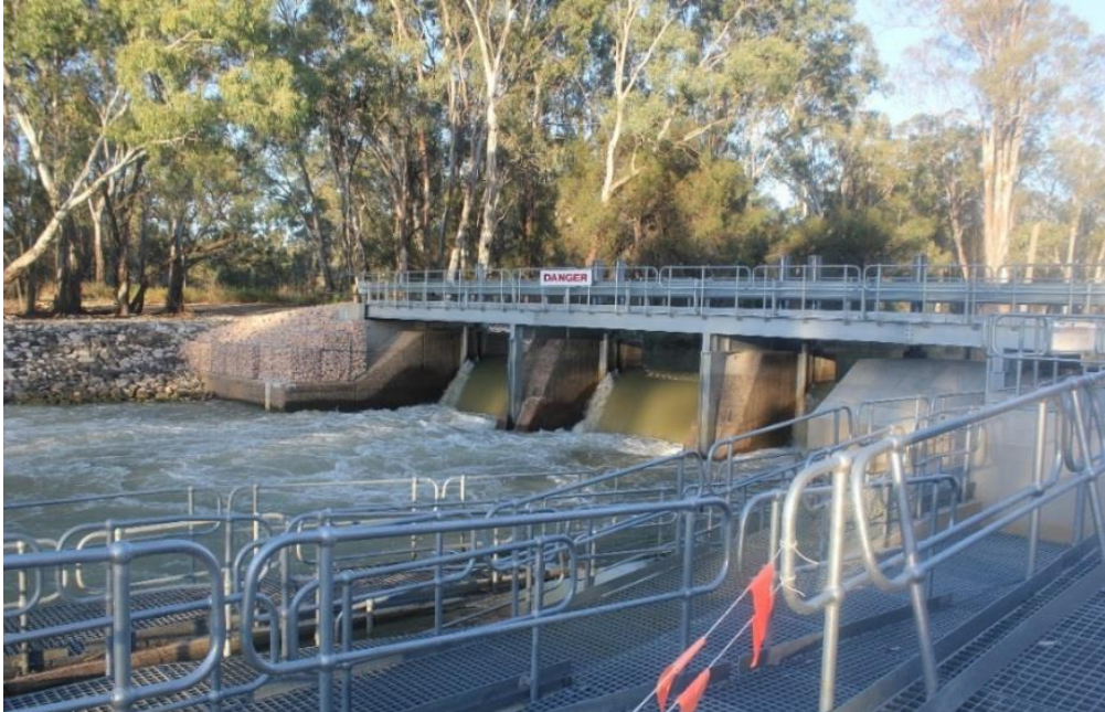
Pipeclay weir in operation during the event
