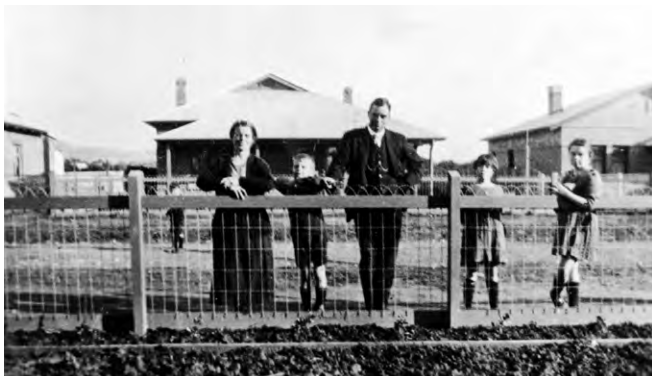
'Moving-in day', to a Thousand Homes Scheme house, Corunna Avenue. Undated photograph. Original held by J. Ball. Source Mitcham Heritage Research Centre.
