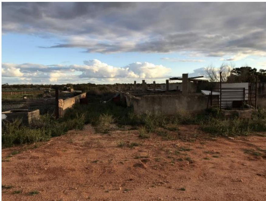
Northern end of the piggery breeding pens showing central corridor
