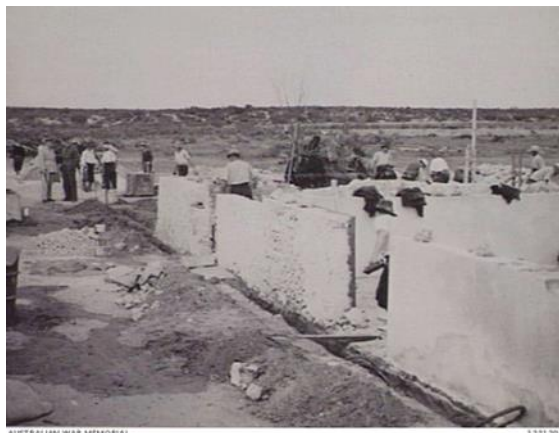
Japanese detainees constructing the breeding pens in October 1943
