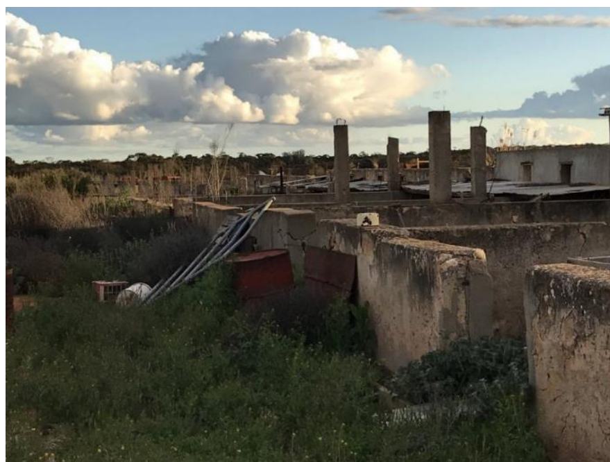
Piggery breeding pens, note the upright supports for the roof
