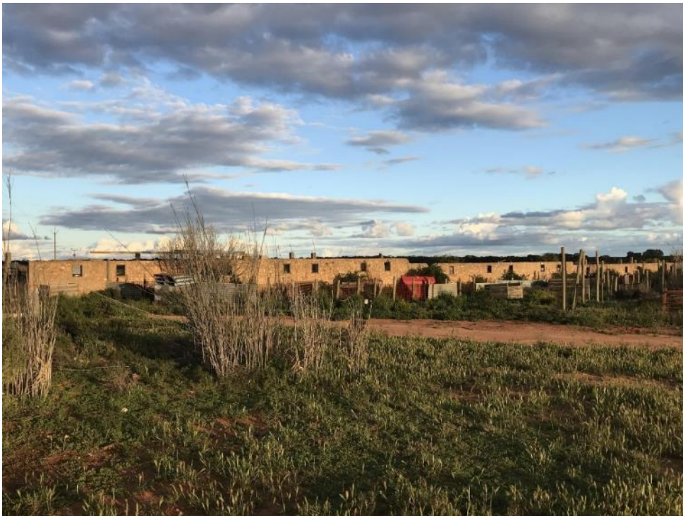
Higher outer (western) wall showing window openings
