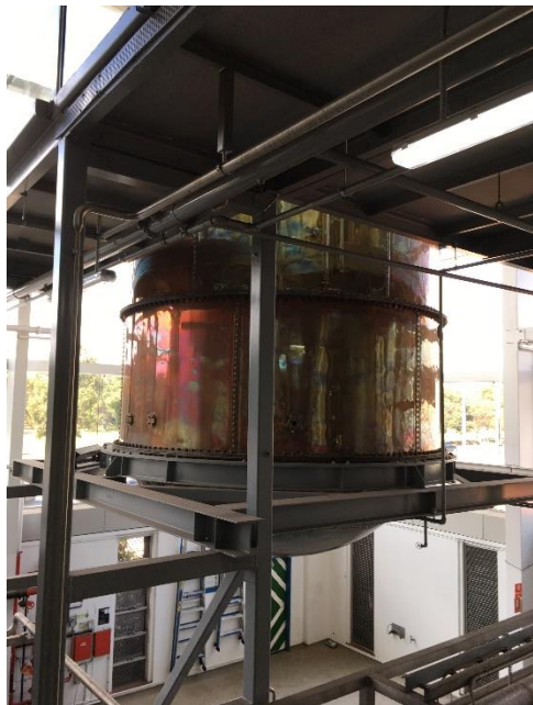
Copper kettle, showing riveting and rounded base.
