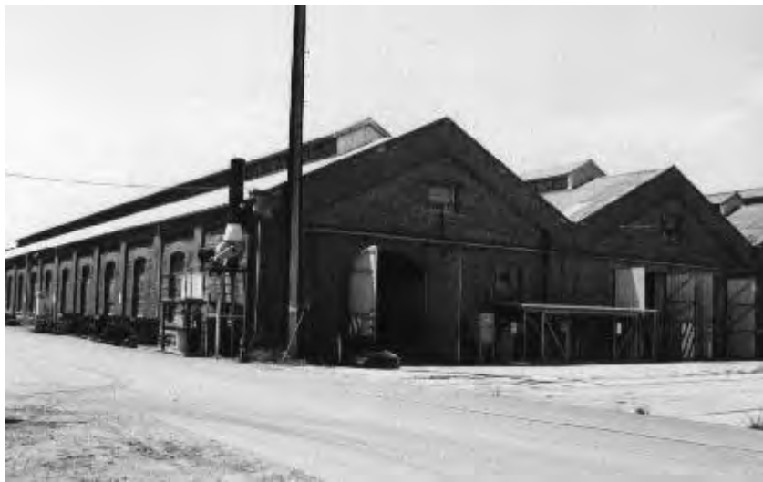
Figure 2. Fabrication Shop SHP 14686
