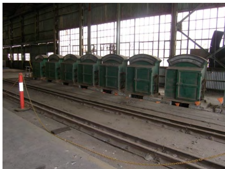
Figure 1. The Weighbridge Platform, Islington Railway Workshops
