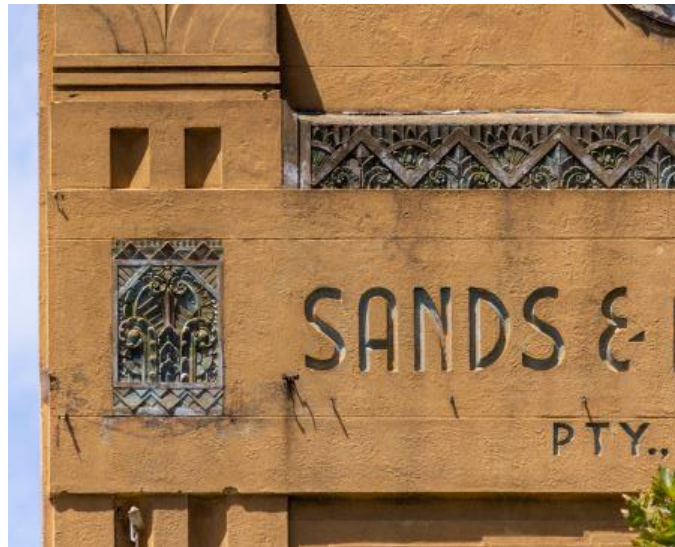
Detail showing the lettering, copper frieze and insert panel at the top of the pilaster
