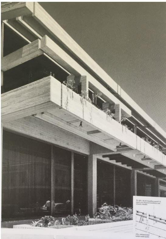
**Associated Securities Limited (demolished) showing the use of off-form concrete**
