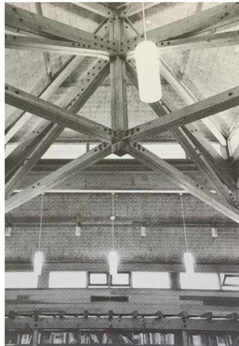
**University of Adelaide Union Building (SHP 17619), showing an example of the brick grille and internal timber framing to roof and 'Solomit' compressed straw panelling to ceiling**
