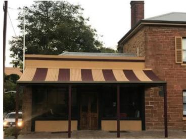
Replace shop awning which covers the footpath in front of the shop. New roof will be will accurately match the existing. The project includes repair of loose stonework and salt damp treatment at the base of the external walls.
