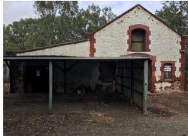
The project includes re-roofing of the coach house which has suffered damage due to leaking of the existing roof and gutters. The external stone walls will be repaired and site drainage improved.
