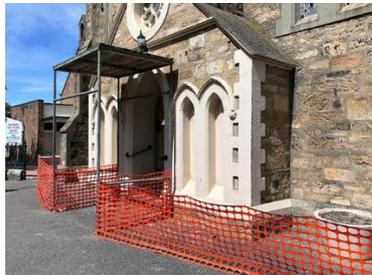
The tower and spire is leaking and has some render which has cracked and fallen from the window and door surrounds. The work will erect scaffolding around the tower and spire, repair structural damage, remove loose render and replacement. The project also includes replacement of damaged metalwork.
