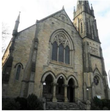
Conservation work is required to the façade of the church. Works include repair to the hooded mouldings over the three pointed entrance arches, salt damp treatment to the bases of the two free-standing columns that support the entrance arches and render to the curving wall to the south end of the entrance steps.
