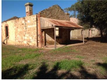
The superintendent's residence has been without a roof as a result of damage due to fire. The re-roofing of the building will prevent further damage and allow further conservation works to take place so the building can once again be used.
