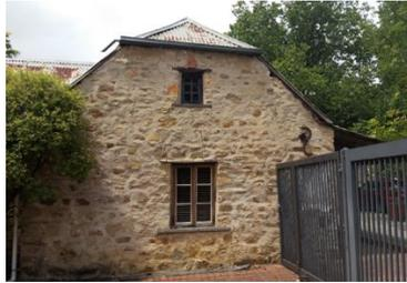
The external walls have been pointed using hard cement mortar. The project will re-point the façade of the cottage using lime mortar.
