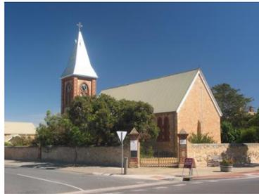
The boundary wall to the church is constructed in red brick and local stone. Boundary walls such as this are important to the public realm and are gradually being lost. The wall is badly cracking and requires repair and some stone replacement.
