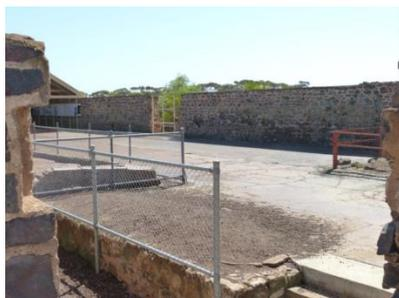
The stone walls at the precipitation works at Moonta Mines are suffering from salt damp and cracking. The project will repair the damaged walls and includes repointing in lime mortar.
