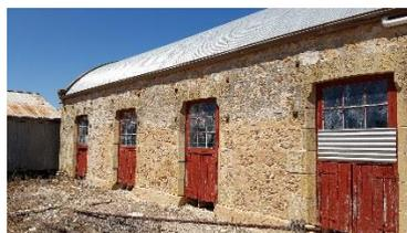
The shearing shed has a dome shaped roof. This is severely corroded and requires replacement. Included in the scope of works is the replacement of the roof and repair of the stone wall.
