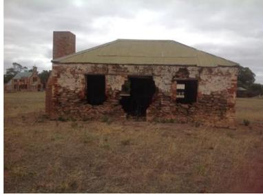
Stabilisation of stone walls by installing a new lintel to the door and windows. Works will secure the building and allow for future conversion for use.
