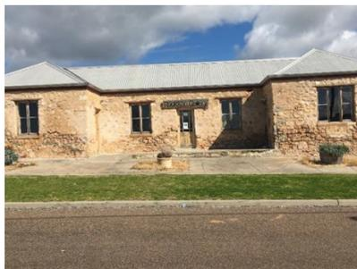
The walls of the gallery have been rendered and pointed using a hard cement mortar. The works include the removal of the cement mortar and replacement with a sacrificial mortar to draw the salts out of the wall. The wall will then be repointed using a lime based mortar.
