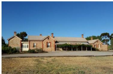
The external walls of the station have some severe cracks and also salt damp damage. The proposed works will repair cracks, repoint walls using lime mortars and reinstate tar damp course. Internally, some walls are also cracked. These will be repaired as part of the project.
