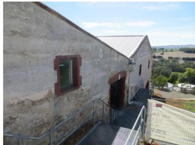
The winery southern wall is an important and highly visible part of this State Heritage Place. It is suffering badly from salt damp and cracking. The project will treat the salt damp and cracking and repoint the wall using lime mortars.
