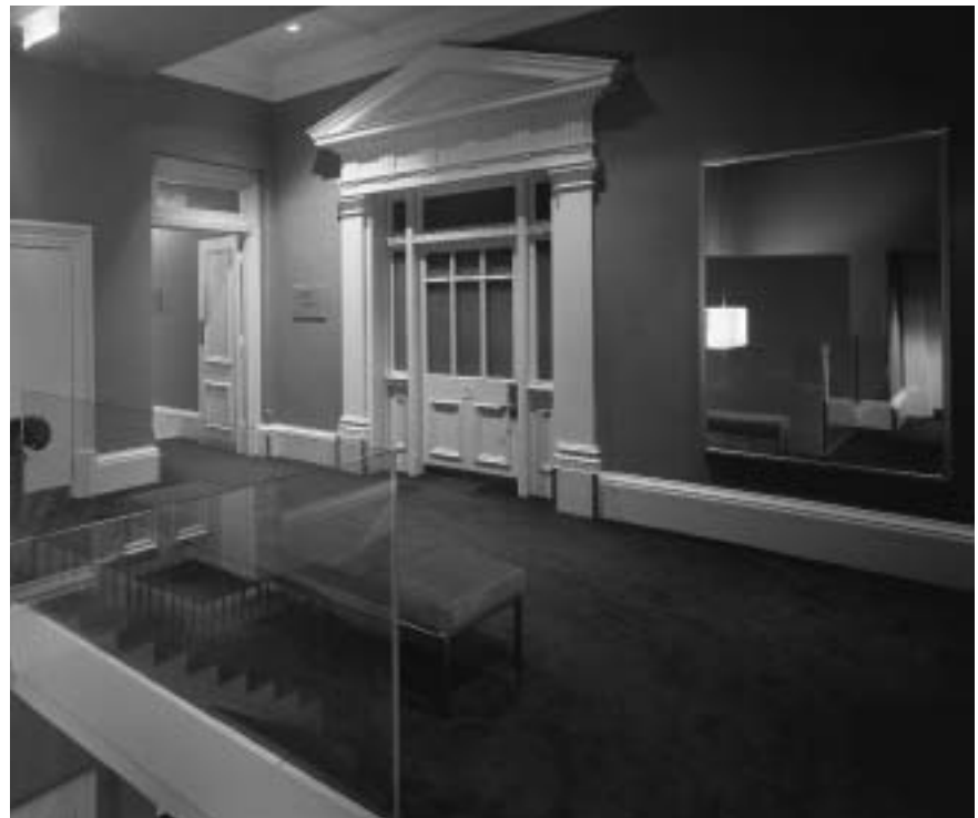
Original ornate door surround revealed during restoration.
