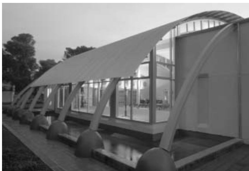
St John's Anglican Church Redevelopment, Salisbury
