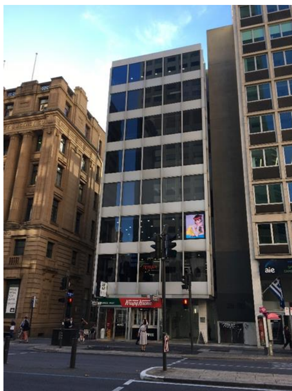
Ferrari House (former Eagle Star Insurance Building) Grenfell St frontage
