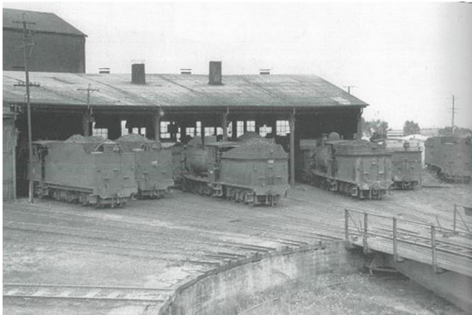
Roundhouse at Port Lincoln Locomotive Depot and Workshops, images taken in 1959, note the multi-pane windows and open front.
