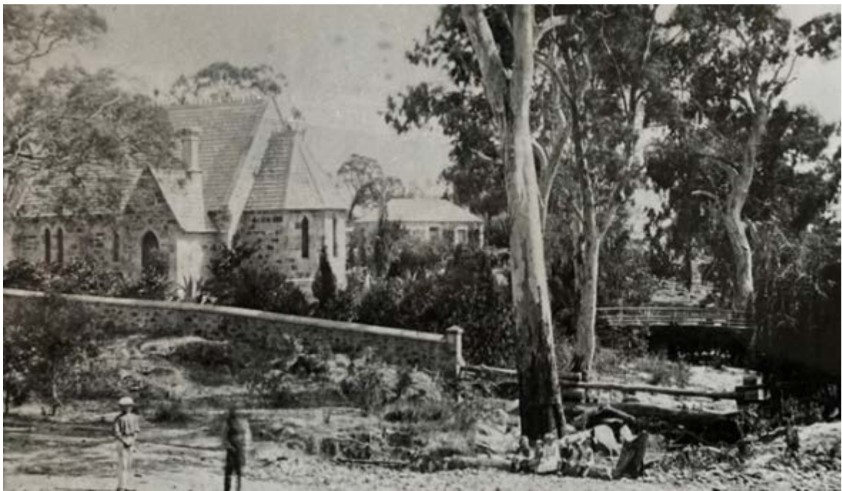
Image: St Thomas' Church Pewsey Vale, image by Capt. Sweet c.1877, note the shingle roof, rector's cottage adjacent to the church and the foot bridge across Jacob's Creek
