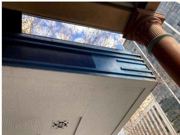
Detail showing the side of the awning
