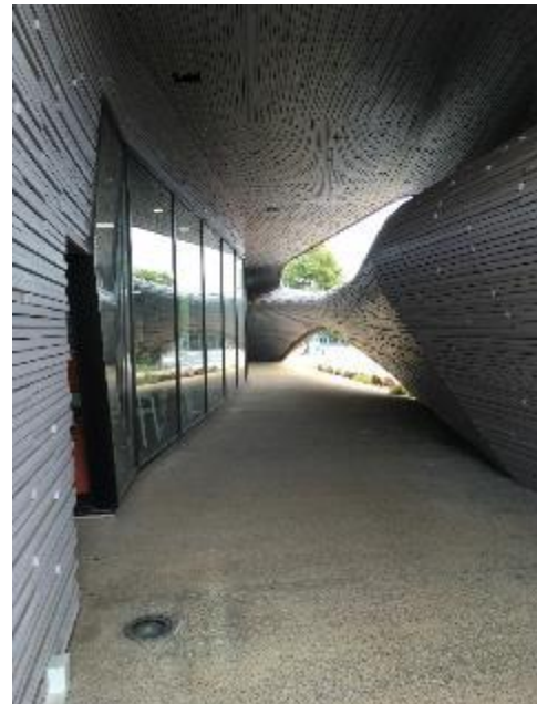
Passageway created down the side of the building by the extruded R. Note the painted timber batons.
