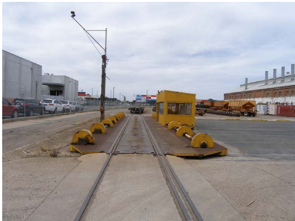
Traverser 1, Islington Railway Workshop, flat-bed machine, view to south, 2017.
