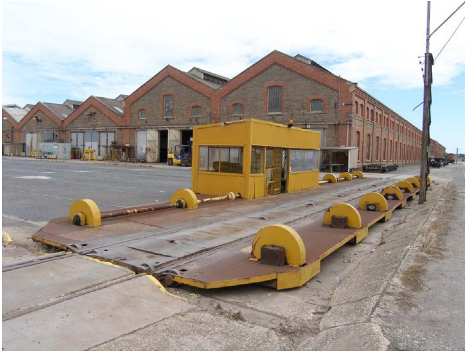
Traverser 1, Islington Railway Workshop, flat-bed machine view to north-west, 2017.
