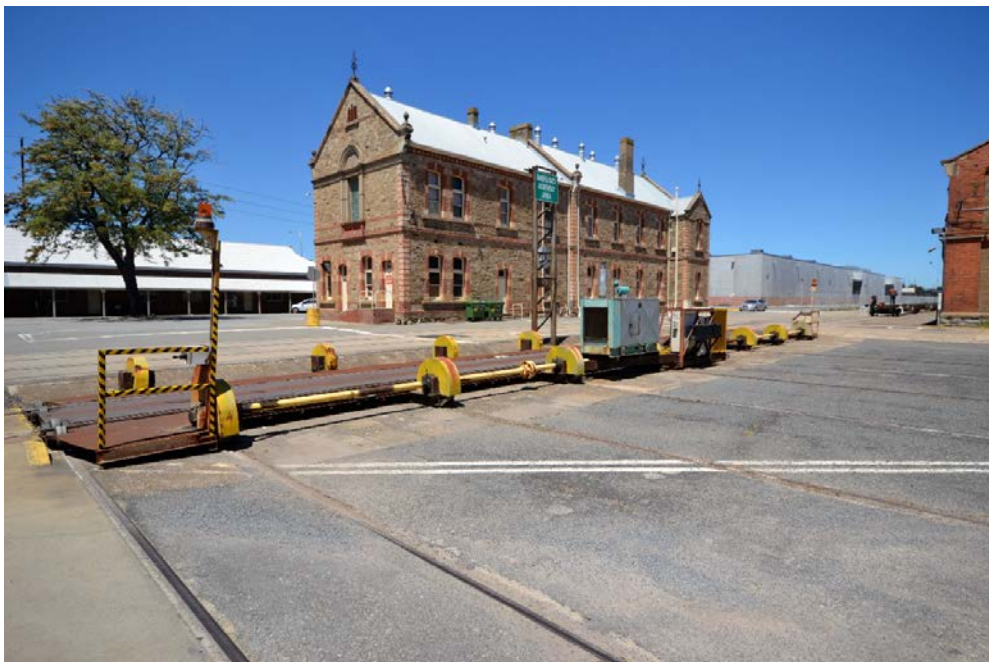
Traverser 2, Islington Railway Workshop, flat-bed machine, 2016.
