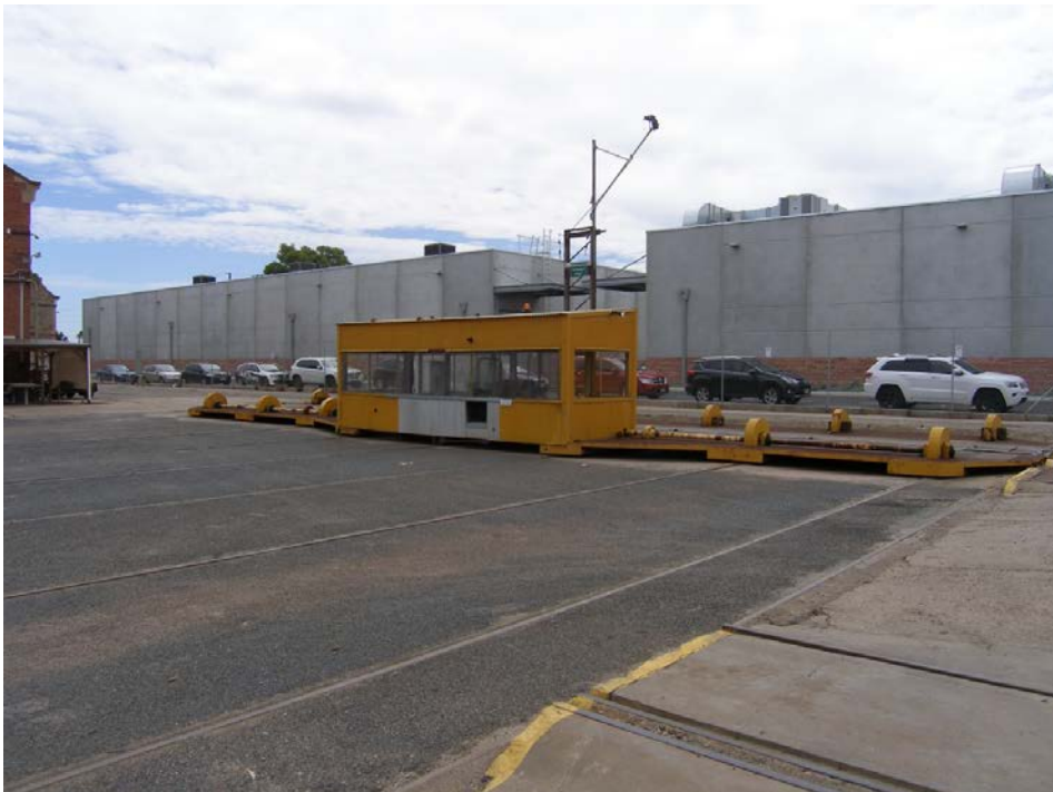
Traverser 1, Islington Railway Workshop, flat-bed machine, 2017.
