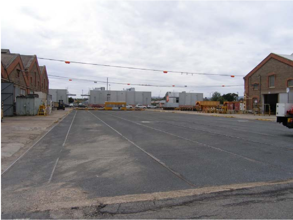
Traverser 1, Islington Railway Workshops, extent of run, looking east, 2017.
