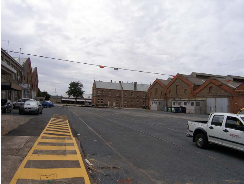
Traverser 2, Islington Railway Workshops, extent of run, looking east, 2017.
