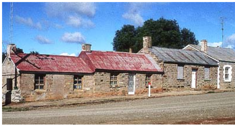
Attached cottages in Truro Street, 2005
