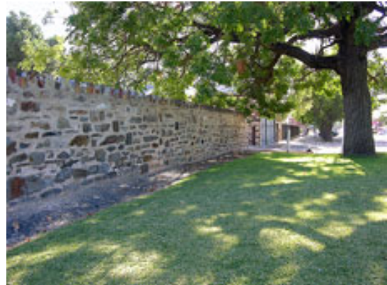
Wall on Commercial Street (west), 2005
