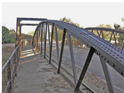
Footpath, Redruth Bridge, 2005
