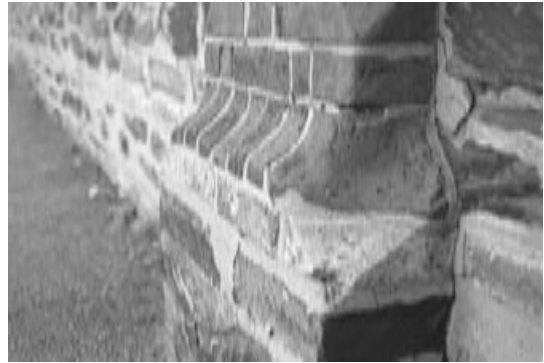
These bricks at the former Grote Street Model School, Adelaide, record the wear of many boys' hobnail boots.
