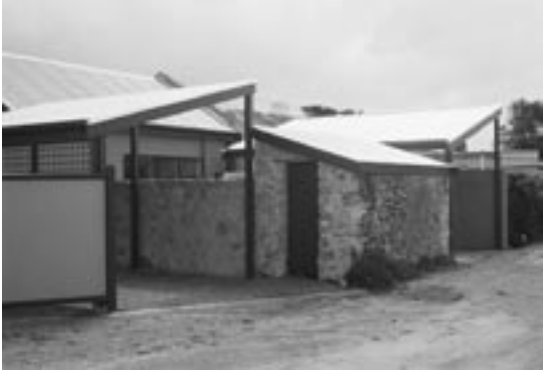
The simple skillion roofs of these new carports complements the original stone outbuilding. Little Scotland, Goolwa.
