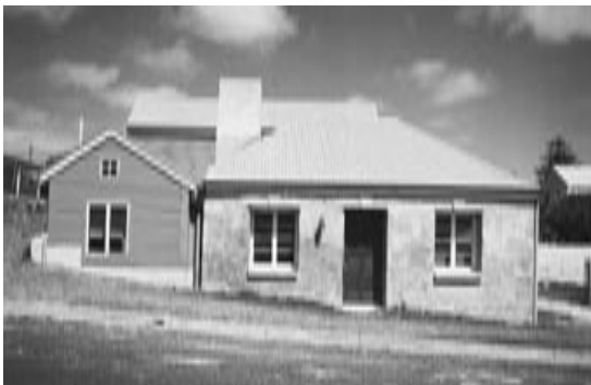
Additions to the Criterion Cottage in Robe have been articulated into small forms that retain the dominance of the original. New materials and windows complement but do not mimic the original.
