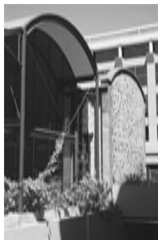
Additions to the Frome Street Stables in Adelaide respond to the traditional form but with modern materials and expression. There is no confusion between new and old.
