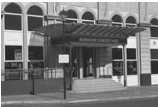
This distinctive new entrance to the Norwood Town Hall has improved access and fire egress. Along with conservation work and new services, this has made an under-utilised hall into a viable, modern concert venue.
