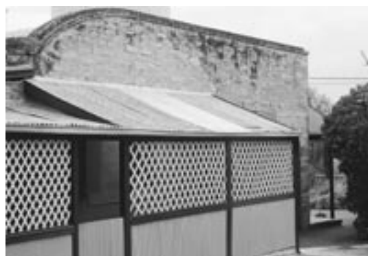
Corrugated polycarbonate roofing provides an unobtrusive skylight.
