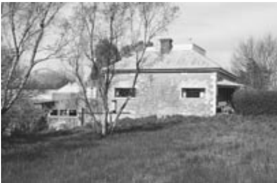
The character of this cottage has been compromised by an unsympathetic roof extension and by new windows that are horizontal rather than vertical in proportion.
