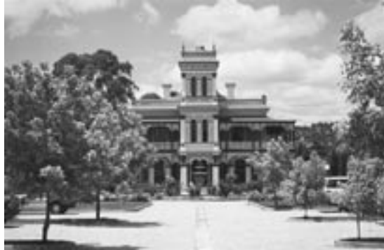
New car parking at Eynesbury College complements the formal character of the building.
