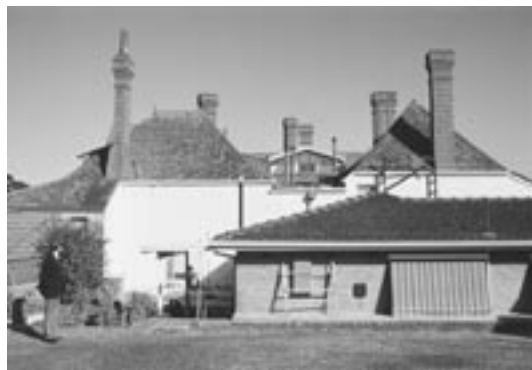
The slate roof and original chimneys of Waite House are inherent design features. The caretaker's residence is not. A roof extension is well concealed behind the main roofs.
