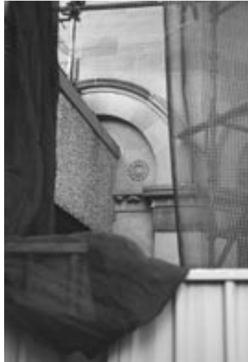
This 1967 addition to the State Library showed little regard for its heritage value. Changed community attitudes would prevent such mistakes today.
