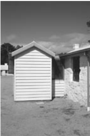
New bathrooms to the rear of the Paxton Square cottages in Burra are separated from the lean-to by a recessed link.
