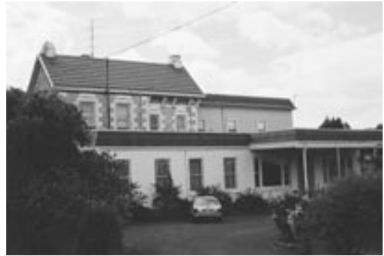
Ad hoc additions and unsympathetic reroofing have largely concealed this house constructed of dolomite.
