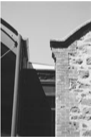
Steel and glass complement but do not imitate the stonework. The new is separated from the old by a recessed link. Frome Street Stables, Adelaide
