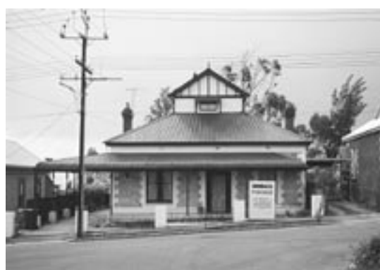
Extending this verandah to form a carport has spoilt the symmetry of this cottage.
