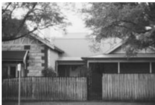
Hipped and gabled extensions of the main roof form.
