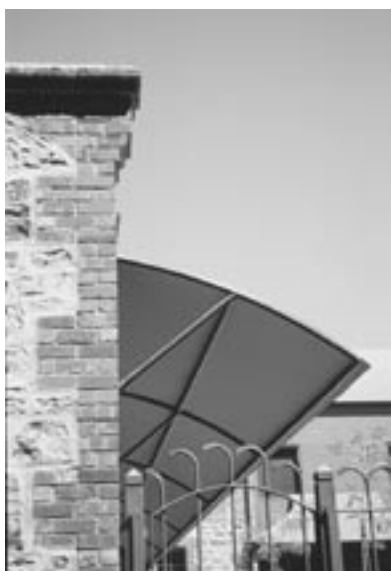
A cleanly detailed cantilever canopy contrasts with the texture and patina of the masonry wall. Frome Street Stables, Adelaide
