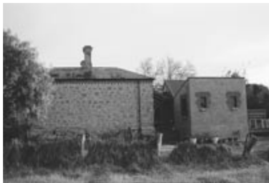
These additions to a stone cottage in Goolwa follow traditional practice and forms but are clearly contemporary.
