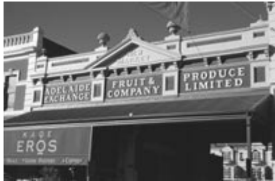
Parapet walls can be used to conceal low pitched roofs. Former East End Market, Rundle Street, Adelaide
