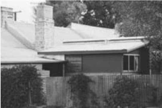
House addition using the existing lean-to as a link.
