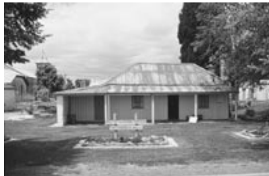
Ulva Cottage in Penola awaits the reconstruction of its fence and cottage garden to complete its restoration.
