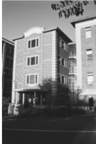
A glazed stairwell has been used to create a setback link for this addition for the CSIRO in Kintore Avenue.
