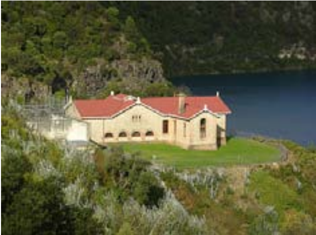
Blue Lake Pumping Station, April 2005
