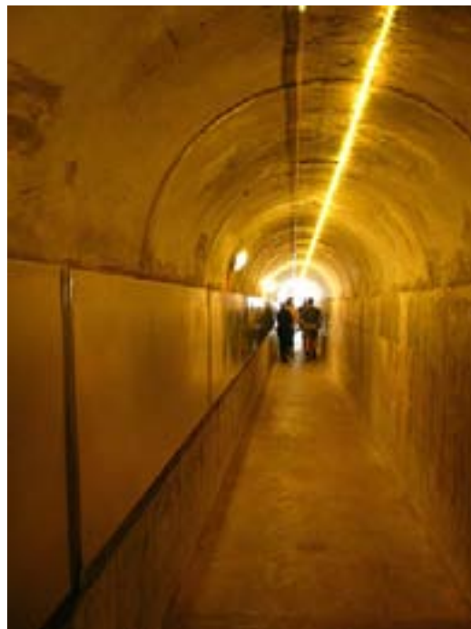
Tunnel leading to the Lake surface, 2005
