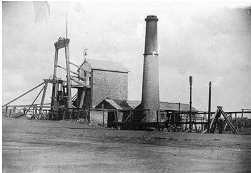
Hughes pumping house at the Moonta Mine 1900 Photo B 58893: State Library of SA
