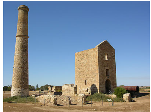
Hughes Pump House & Chimney, 2005
