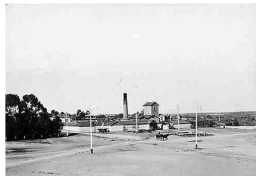
Hughes Pumping Plant 1916 Photo B 9207: State Library of SA
