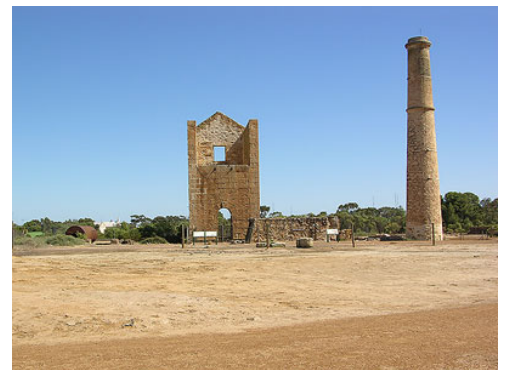
Hughes Pump House & Chimney, 2005
