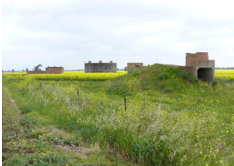
Concrete filling platform, September 2007
