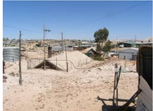
Roof of original building, 2006
