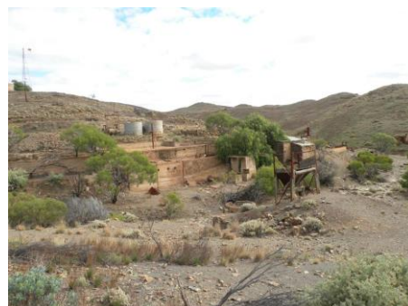
Prince Alfred Copper Mine Precinct, via Cradock - View to north west [1970s leaching plant, showing concrete tri-level layout.] (DSCN 1990 P. Bell)
