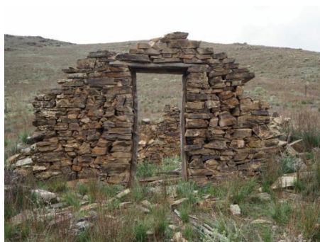
Prince Alfred Copper Mine Precinct, via Cradock - View to north east [House or pub ruin in township.] (DSCN P42490111 J. McCarthy)
