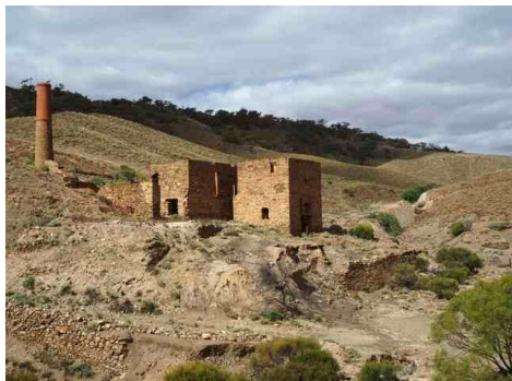
Prince Alfred Copper Mine Precinct, via Cradock - View to south east [Crusher house (right), engine house (centre), boiler house (left) with chimney and flue at rear and remnant drystone walling and tailings in foreground.] (DSCN P42490059 J. McCarthy)
