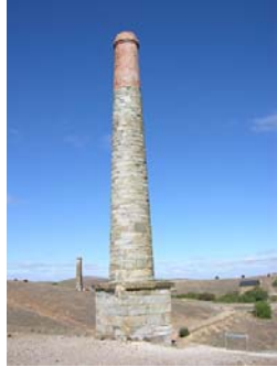
Cornish Crusher Chimney, 2005
