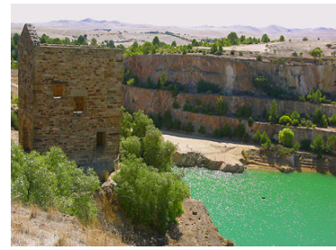
Graves Pump House, 2005
