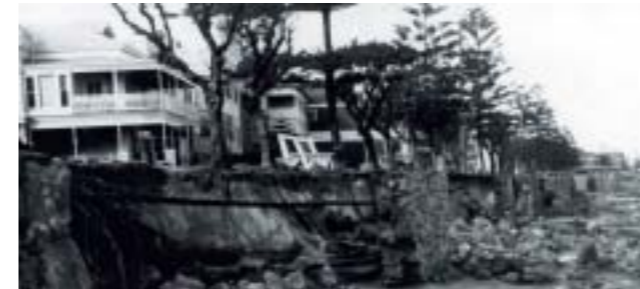
Storm damage at Glenelg, 1960
