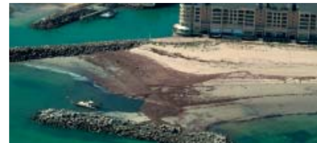
Dredging of sand and seagrass at the Glenelg harbour
